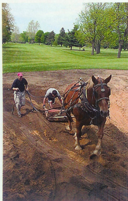
Construction the Golden Age way
